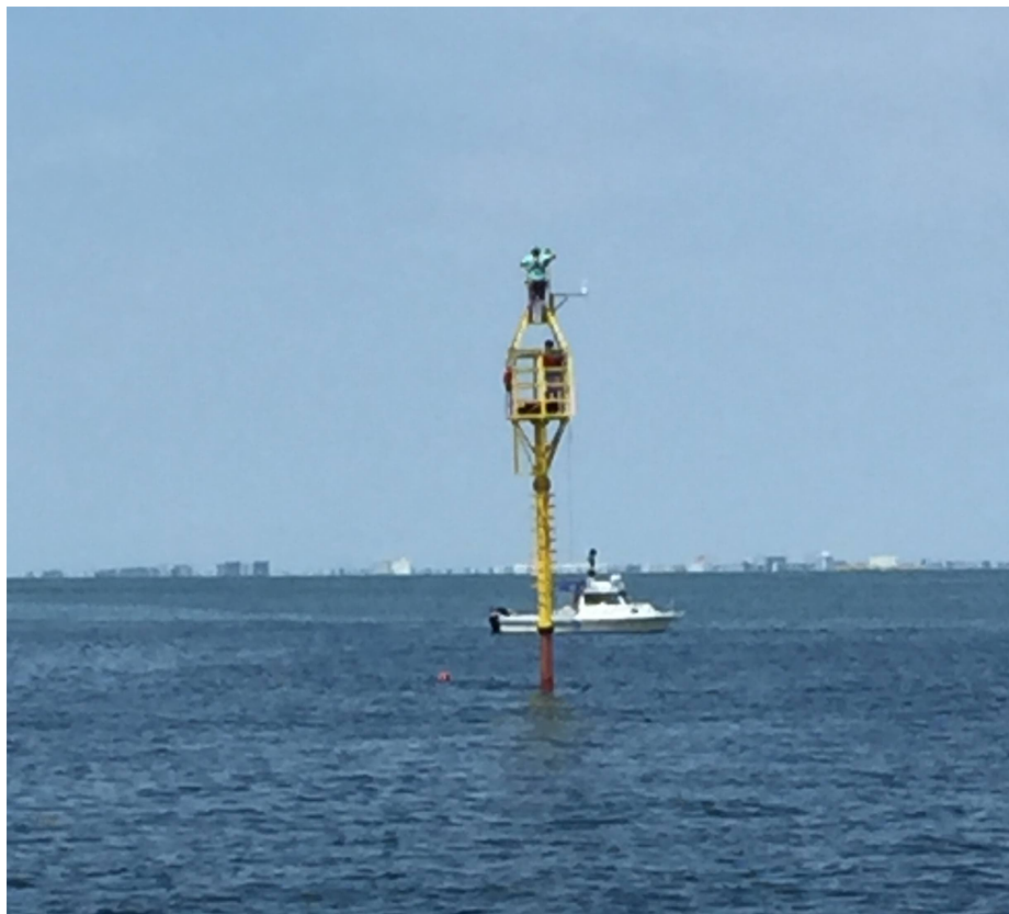
Figure 16. Jay Law installing the GPS antenna on the highest point of the buoy.
