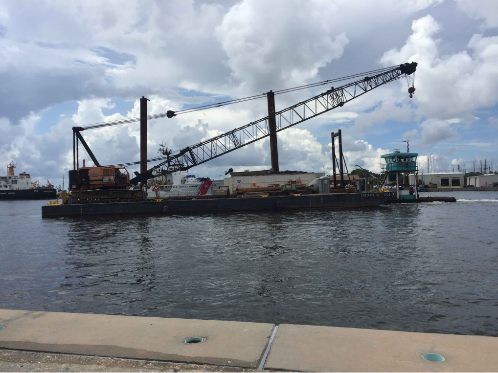
Figure 12. Barge approaching sea wall for loading operations.
