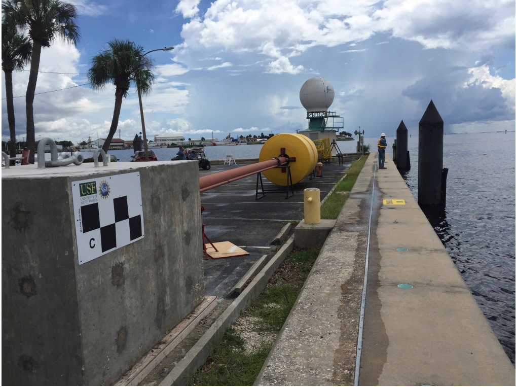
Figure 11. Buoy and ballast on sea wall prior to loading.
