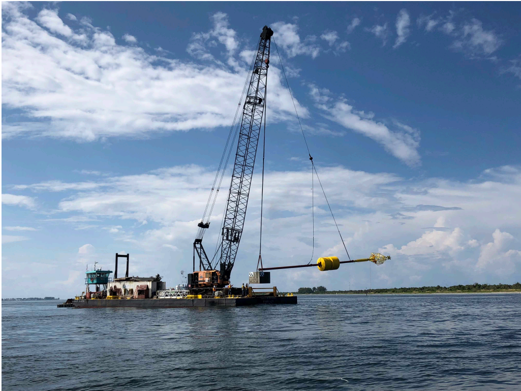
Figure 14. Two views of the barge deploying the buoy.
