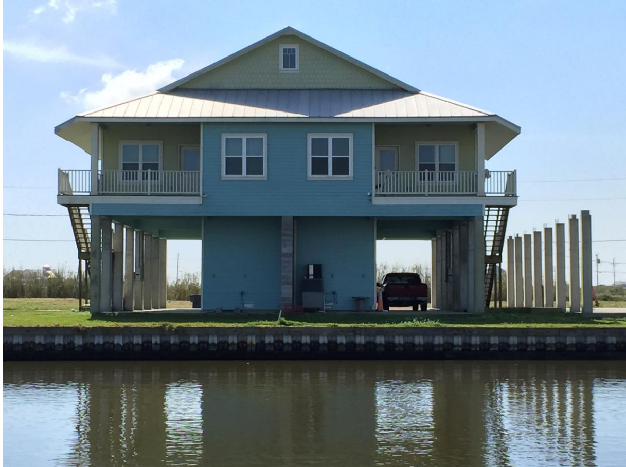
Figure 7.3. A delta house, with the main living space on the second floor. Photo by the author, taken March 2016.
